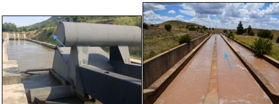
Figure 2. The LUSIP sand trap (LHS) and the Tienfontein settler (RHS)
