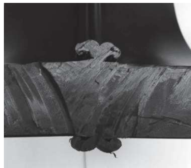
Fig.1 Weld bead projection of pipe d355x32,2 SDR11 PE100
